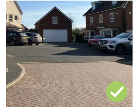
Figure 83: Paving is used at Gladstone Place to highlight the priority of pedestrians over vehicles.
