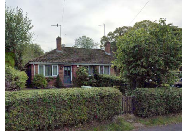
Figure 33: 1-storey bungalow on Sculthorpe Road
