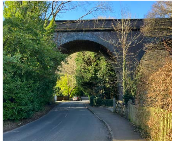
Figure 08: The railway bridge on Churchill Lane
