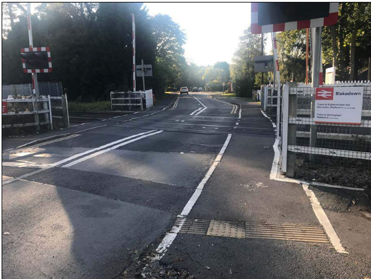
Figure 1.3: Photograph of Level Crossing in Blakedown
