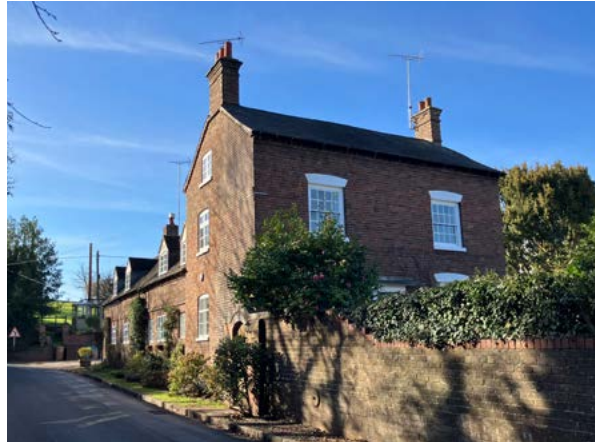
Figure 31: Two-storey house and cottage facing the street in Churchill
