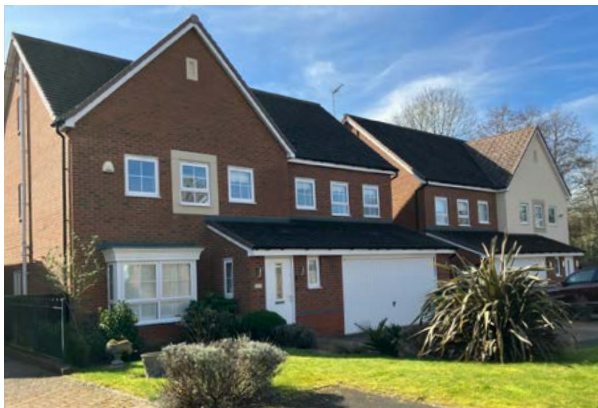
Figure 30: Typical detached house at Gladstone Place
