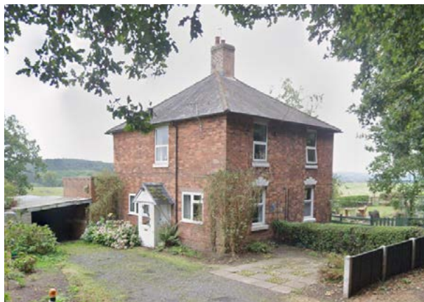
Figure 60: 2-storey house in Area 4
