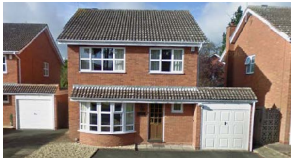
Figure 48: Red brick detached house on Mill Close
