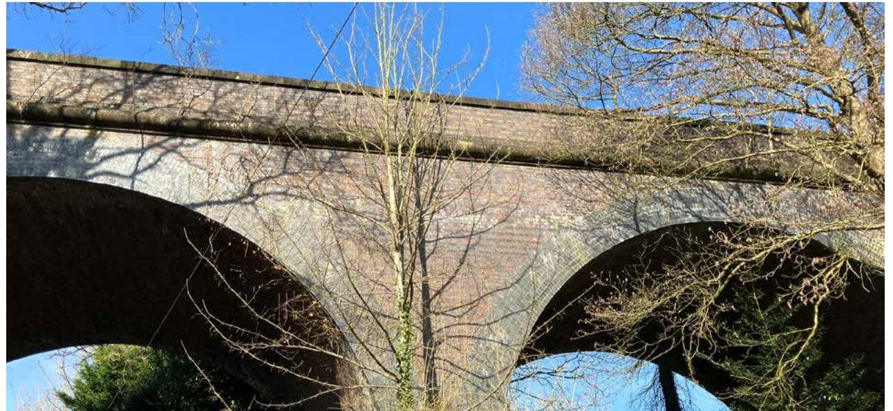
Figure 17: Churchill Lane railway bridge
