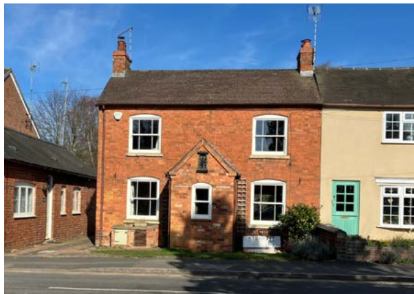
Figure 41: Red brick cottage on Belbroughton Road
